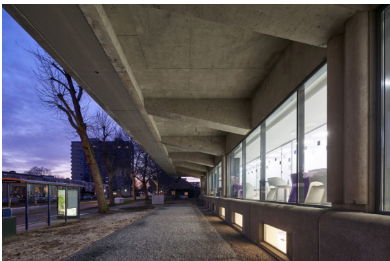
Figure 93. Structure - street level
