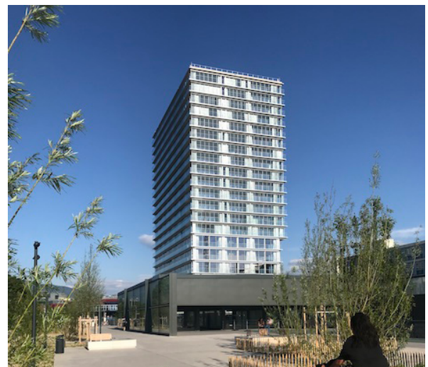
Figure 56. Tour Opale - Completed
