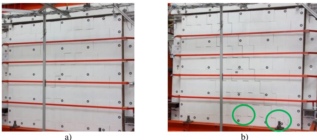
Figure 5.58 a) Formation of stairstep cracks and b) cracks in the blocks at 2.1% of drift
