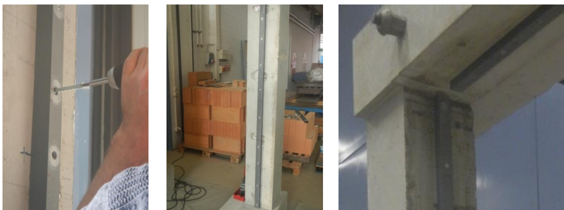
Figure 3.6 Placing plastic bars at the columns and the upper beam
