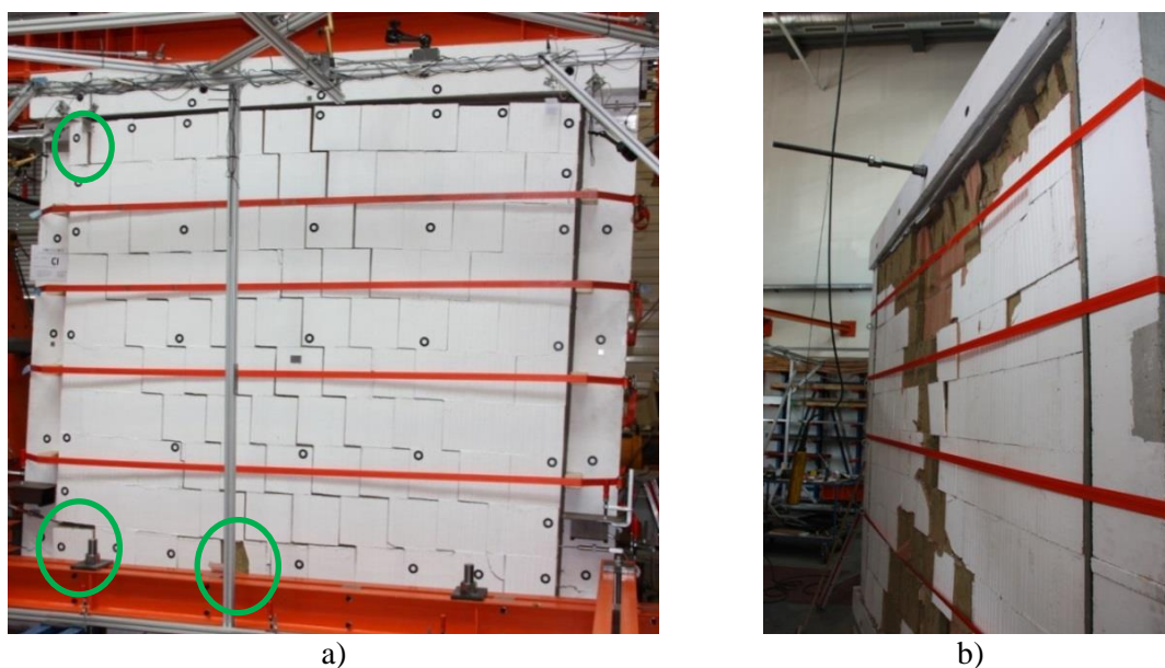
Figure 5.63 a) Cracks in the wall and b) damage of the backside of the wall at the end of Test CI
