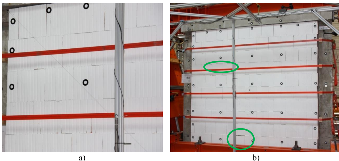
Figure 5.31 a) Opening of bed joints and b) stepwise cracks in compressed diagonal and cracks in the bricks
