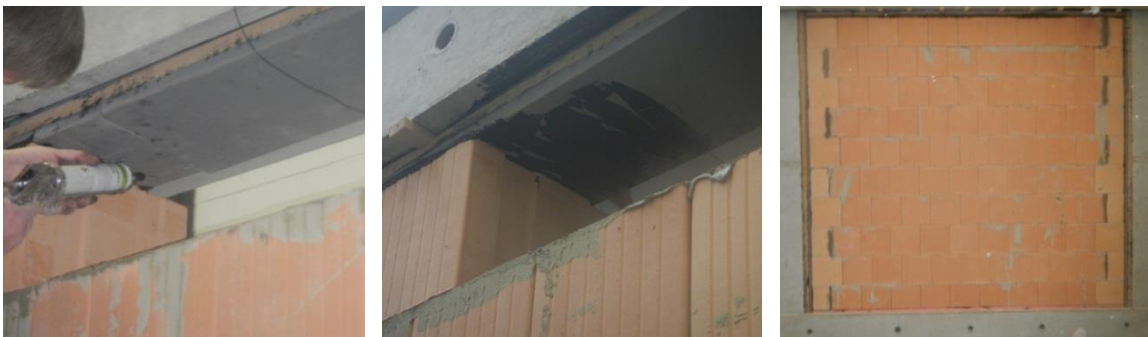
Figure 3.11 Gluing the last row and finalized wall
