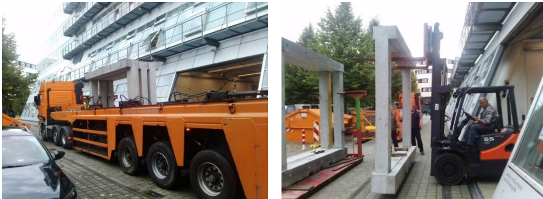
Figure 5.6 Transportation and delivery of the RC frames
