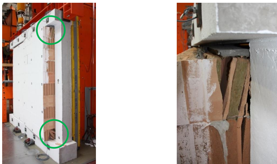
Figure 5.27 Local failure of the bricks at the top and bottom of the wall at the end of the Test BO
