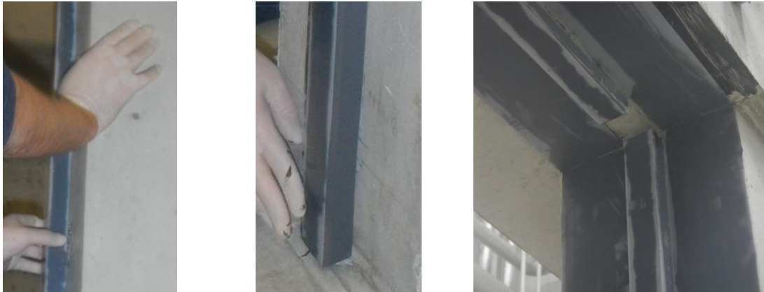
Figure 3.7 Applying a sliding surfaces on the plastic bars
