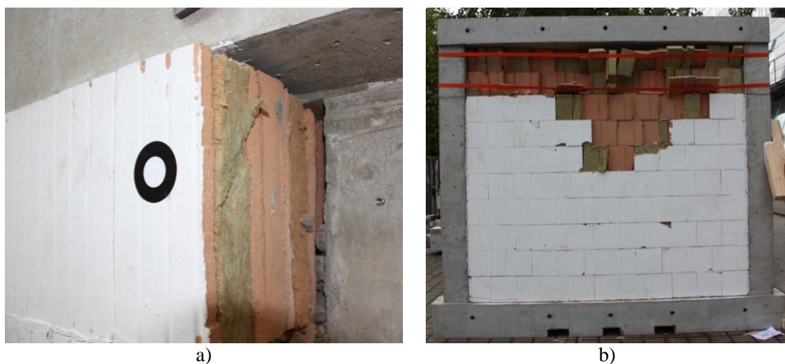
Figure 5.40 a) Failure of the brick in the upper corner of the wall and b) damage of the backside of the wall at the end of the whole loading protocol
