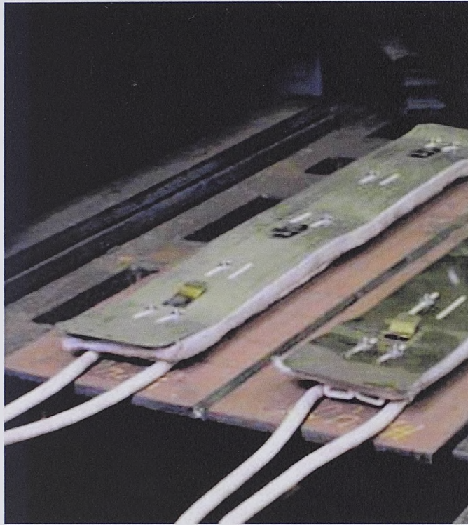
Figure 4.14 Electric preheater elements around the prepared joint. [70]
