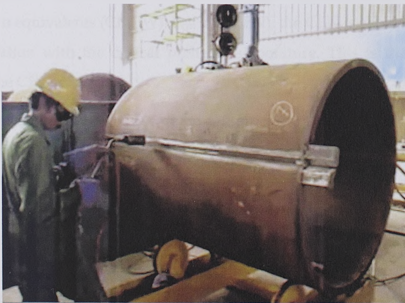
Figure 4.15 Single nozzle gas burner preheating of long seam pipe. [71]
